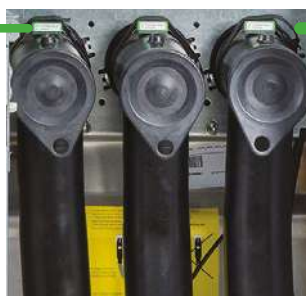
TH110 mounted on cable termination
