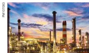
Separate MV consumer substation
