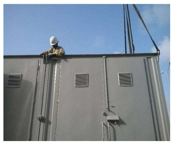
26. Apply the cementex solution on the Sealing rubber and join it with the upper corners of Kiosk units.
