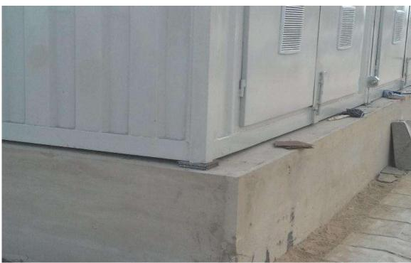
18. Apply the cementex solution on the Sealing rubber and join it on the other Corners of Trafo unit.
